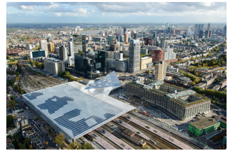
sleutelproject r'dam centraal station
