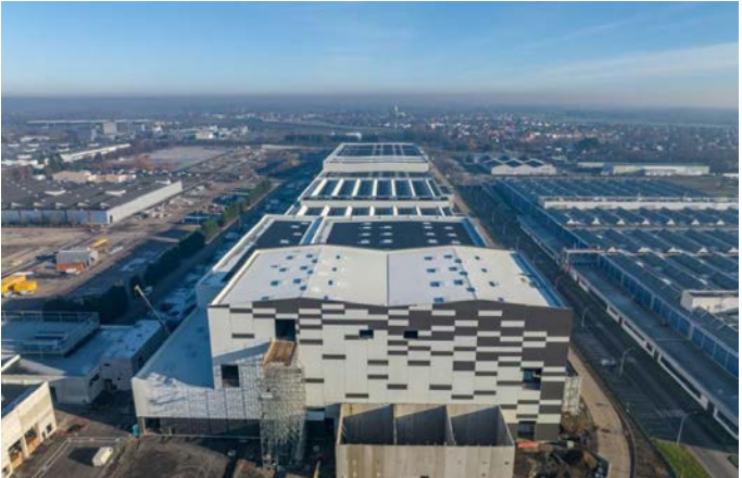
Gigafactory van Automotive Cells Company in Billy-Berclau Douvrin (Hauts-de-France).
